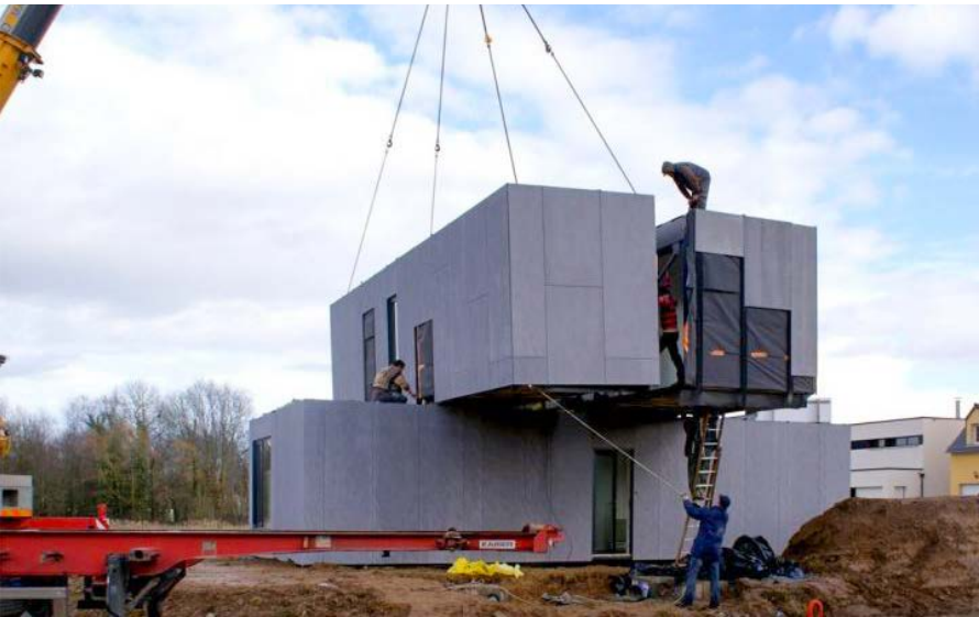
Modular construction of housing reduces the time required to build single- and multi-family housing by up to 50% which reduces overall costs to developers. KOMA MODULAR CONSTRUCTION
