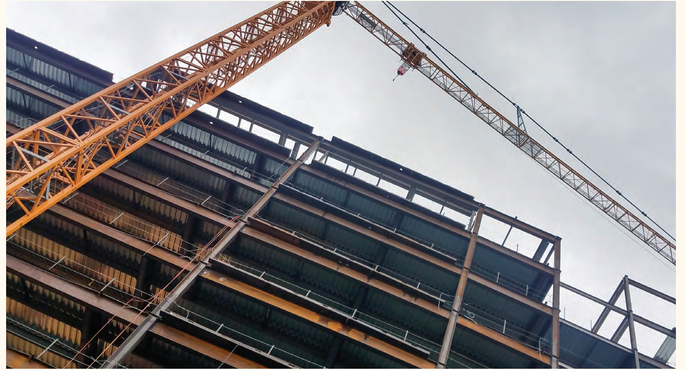
View of new vertical construction. Lauren Corn
