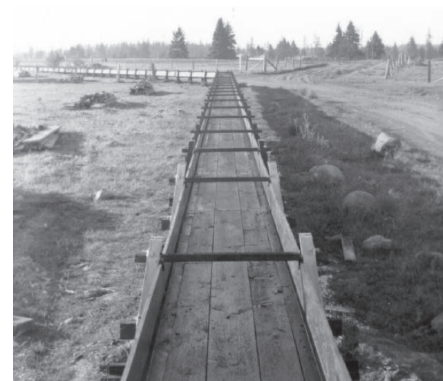
Left: Before underground plumbing, modern water wells, and Tacoma's municipal reservoir at Alder Lake, above-ground wooden flumes, like this one pictured in Yelm in 1935, transported the city's water supply. Drinking water flowed from Spanaway Lake to downtown through these conveyances until 1905, when Tacoma developed a system of underground pipes. TACOMA PUBLIC LIBRARY NORTHWEST ROOM
