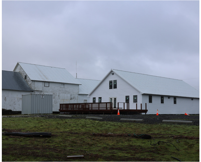
Figure 17: Current building conditions
