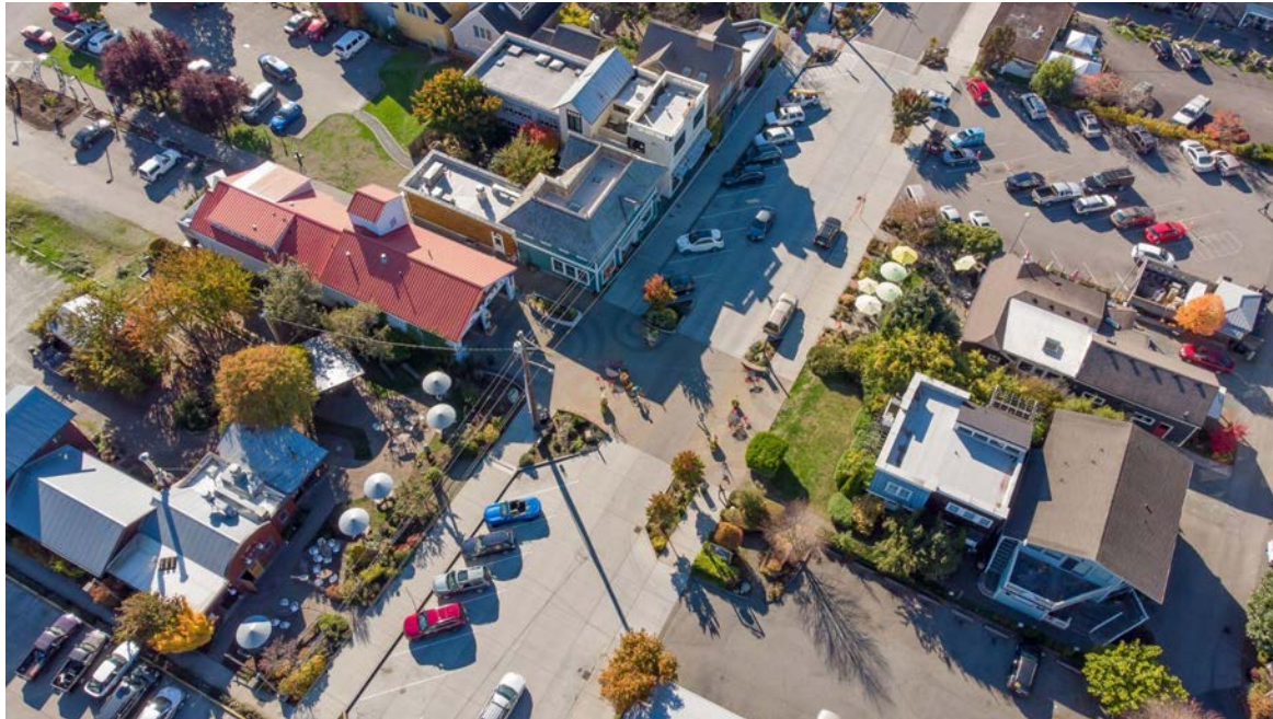
Figure 11. Langley, Washington's Completed Second Street Project (Source: Framework Urban Design).
