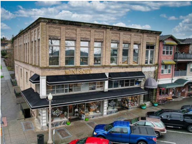
Figure 34. The Marks Building. (Source: Workman Real Estate Services)
