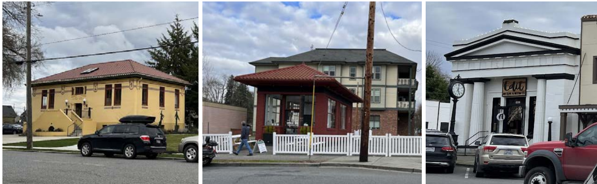
Figure 8. Carnegie Library Building, 802 First Street, and First National Bank, left to right (Photos by Katherine Magee, taken February 7, 2024)
