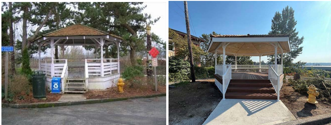
Figure 10. Snohomish’s First Street Gazebo Pre/Post-Renovation Photos. (Source: City of Snohomish Washington)
