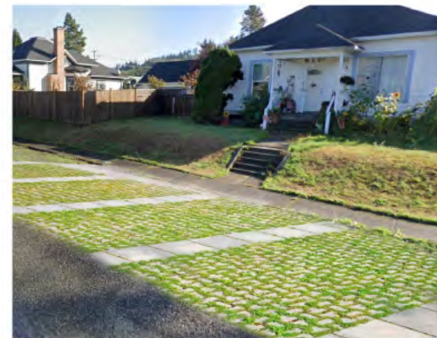
Figure 28: Pavers for unpaved street shoulders
